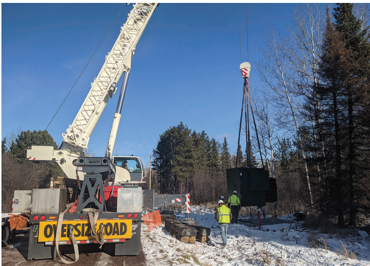
A crane sets a 3-phase step-up/down transformer on the Laine Road during the last phase of an upgrade project in Clover Valley.
